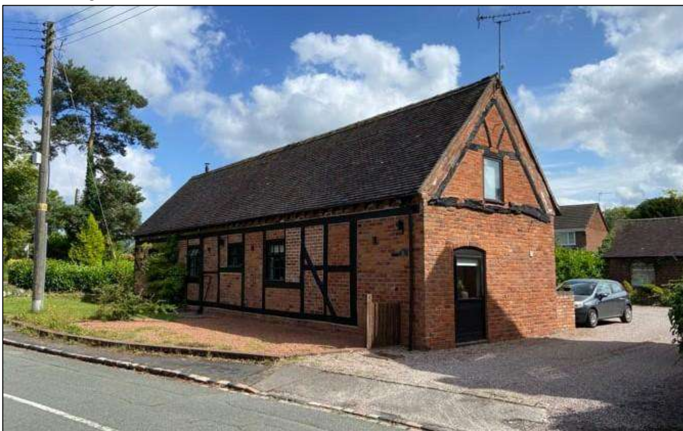
Figure 8 - The Barns, Yarnfield: Grade II listed building
