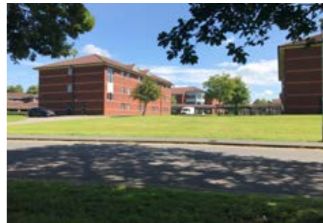
Figure 33: View 9: Existing accommodation blocks
