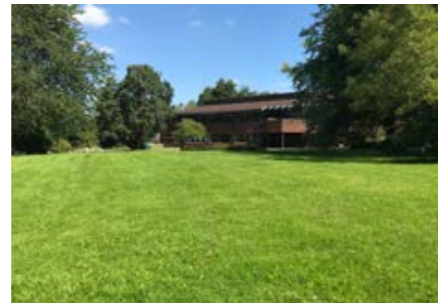
Figure 34: View 10: Existing entrance for office buildings
