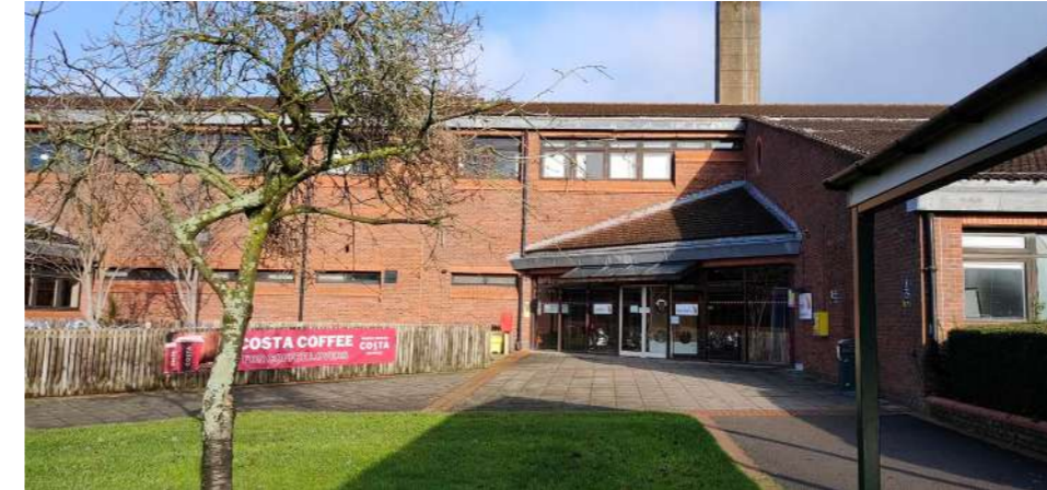
Figure 33: Yarnfield conference centre entrance
