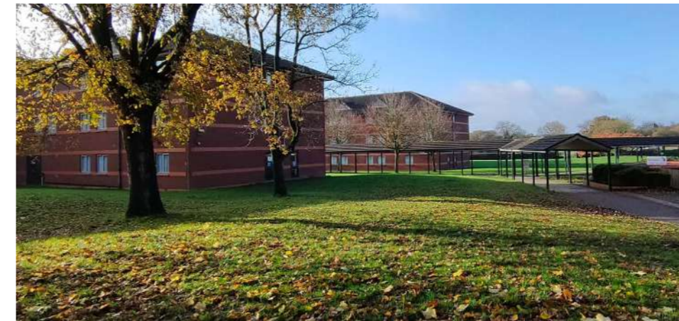
Figure 34: View of accommodation buildings for Yarnfield conference centre
