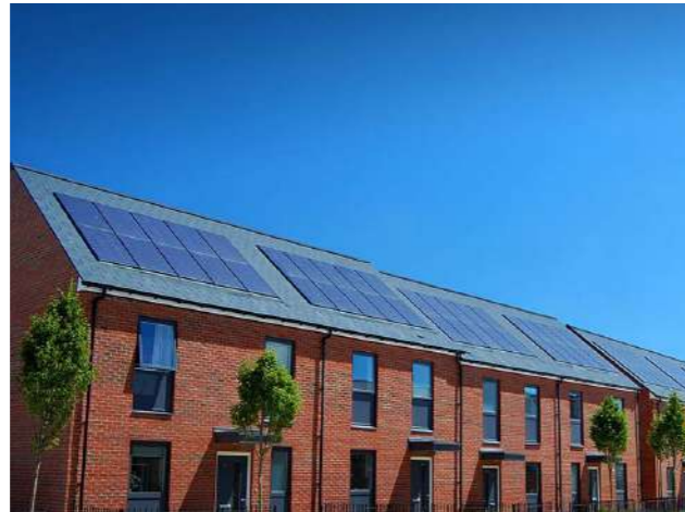
Figure 64: Precedent image - example of integrated solar panelling
