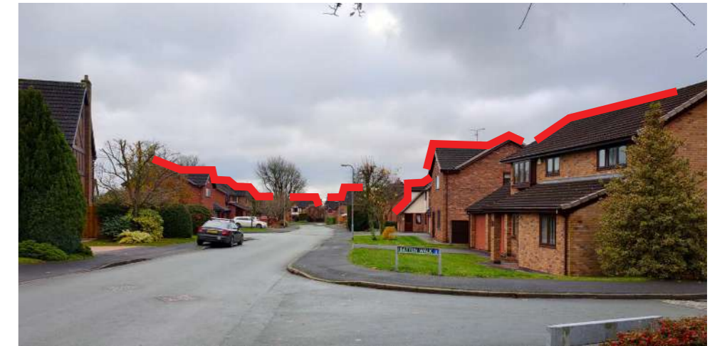
Figure 50: Varied rooflines example within Yarnfield and Cold Meece
