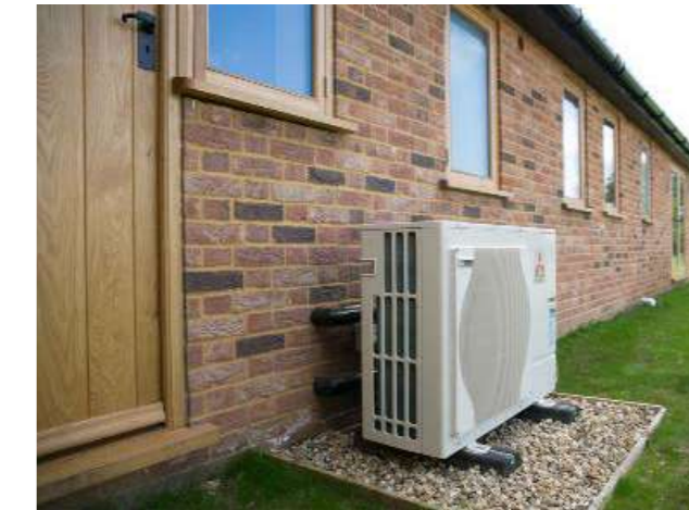
Figure 72: Air source heat pump unit located to the rear / side elevation of a dwelling, so to avoid its visual impact on the dwellings frontage and wider streetscape
