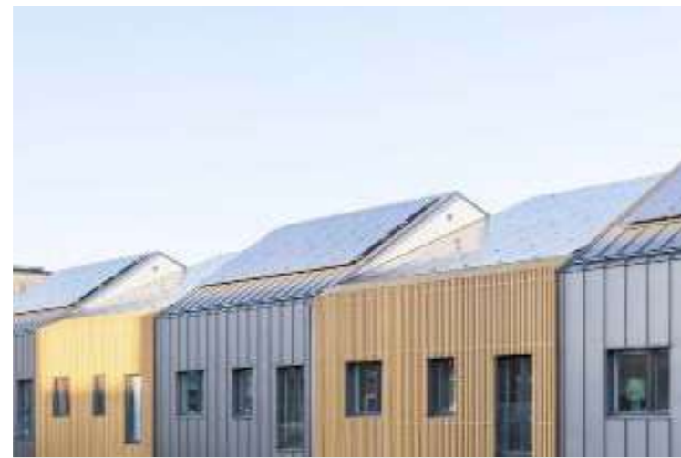
Figure 69: Carefully angled solar panels that harness every moment of the sun
